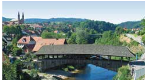
Holzbrücke in Forbach ▶
